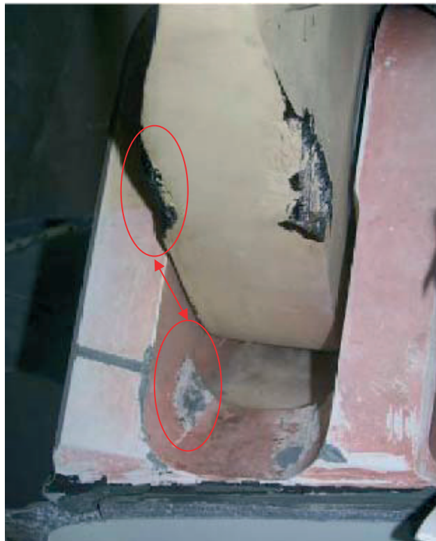
Rear view of the left-hand aft lug: there were marks showing a backwards pivoting of frames 86 and 87
