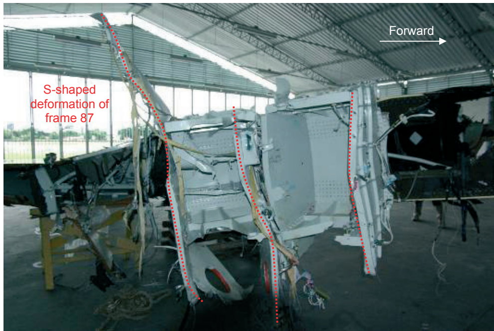
Frames 84 to 87: S-shaped deformation of frame 87, with frames 84 and 85 pushed in backwards
