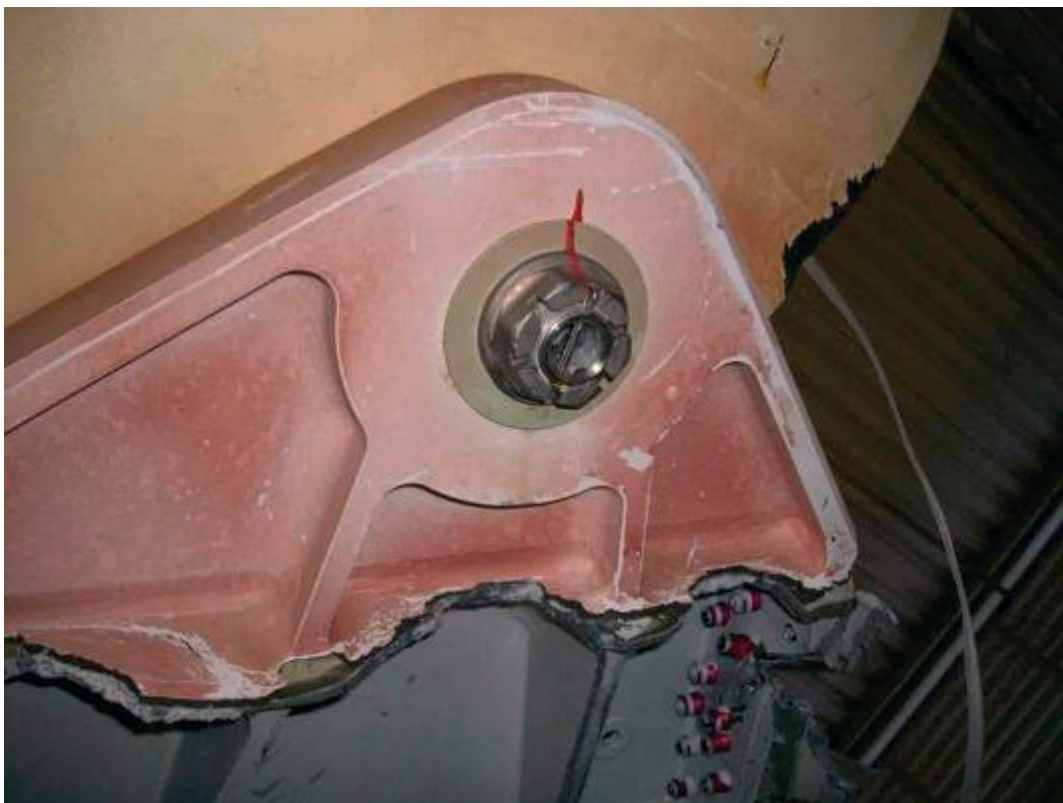
Right-hand aft lug: shearing of the fuselage along main frames 86-87
