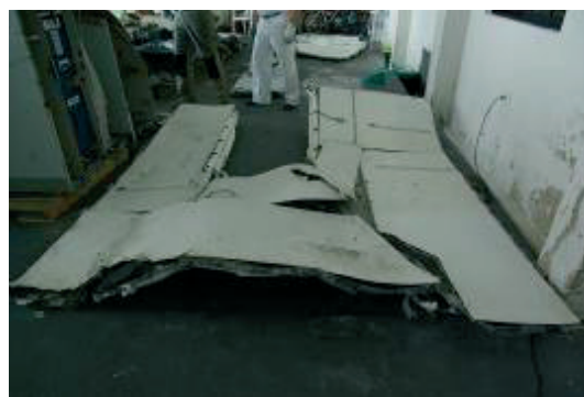
Ceiling of the LDMCR: with top-downwards deformation
