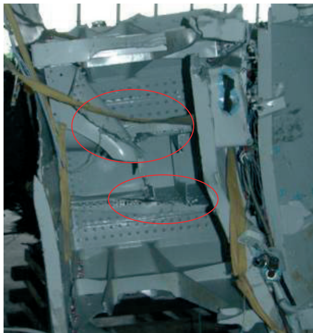
Frames 86 and 87: failure of the horizontal stabiliser actuator supports
