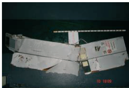
Toilet door (L54) metallic stiffeners deformed by buckling
