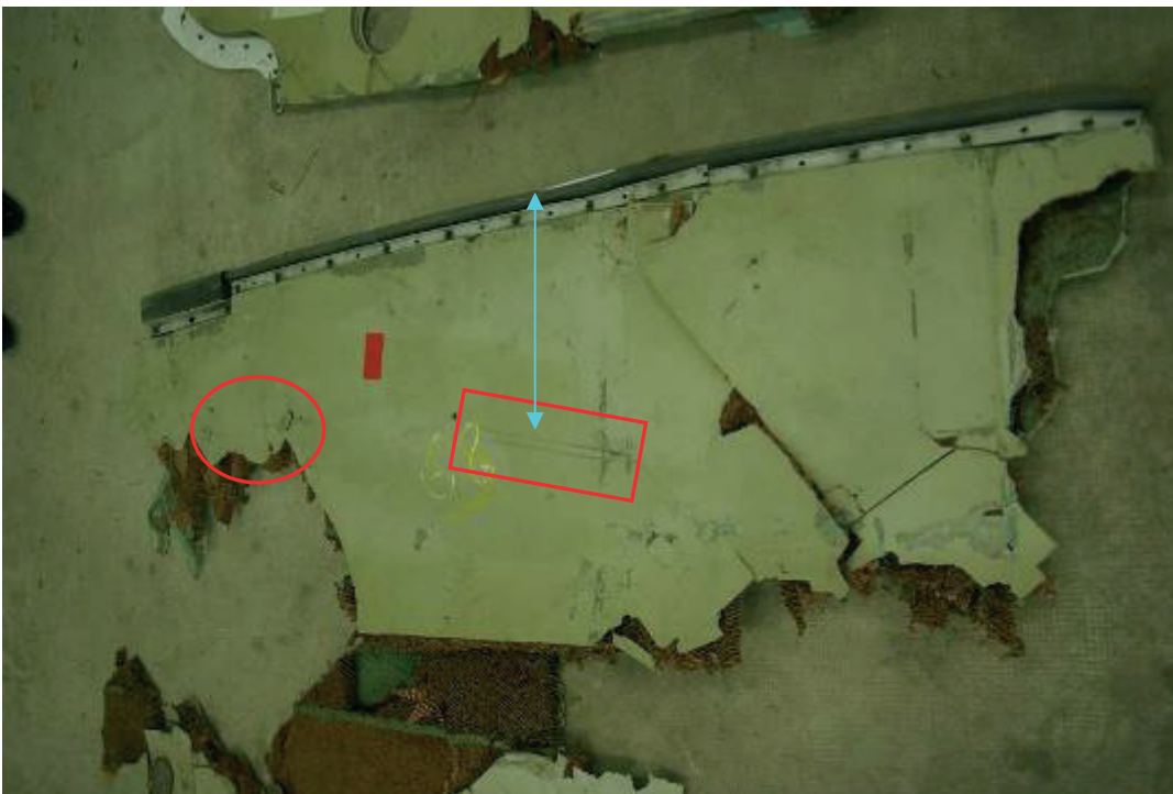
Part of the No. 3 flap track fairing on the left wing
